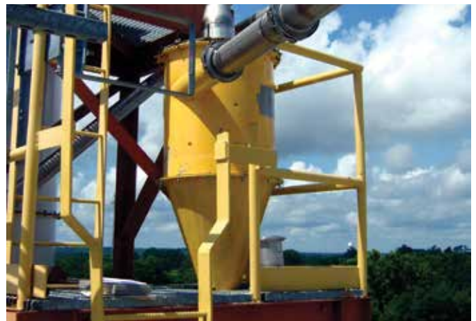
Cyclone clad with Kennametal infiltration braided tungsten carbide wear protection.
