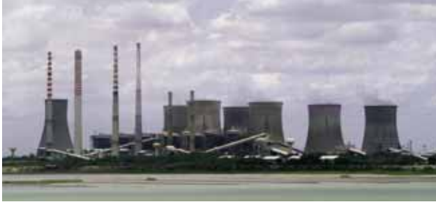
Raichur Thermal Power Station — Raichur, India
